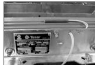
Fig. 4 1 or 2 PT100 on the core
