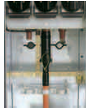
Connection detail: EUROMOLD (K-152SR) plug-in elbow connector
