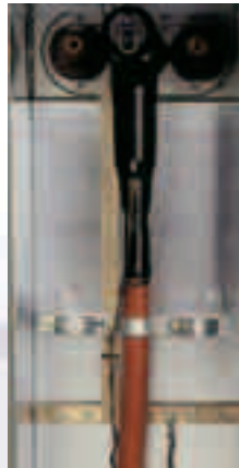
Connection detail: EUROMOLD (K-400TB) screw-mounted elbow connector
