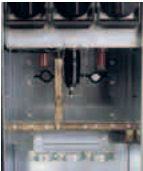
Connection detail: EUROMOLD (K-158LR) plug-in elbow connector
